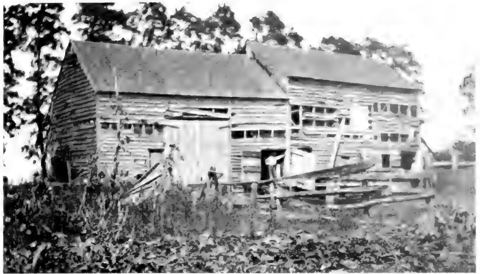
Another View of the Barn
